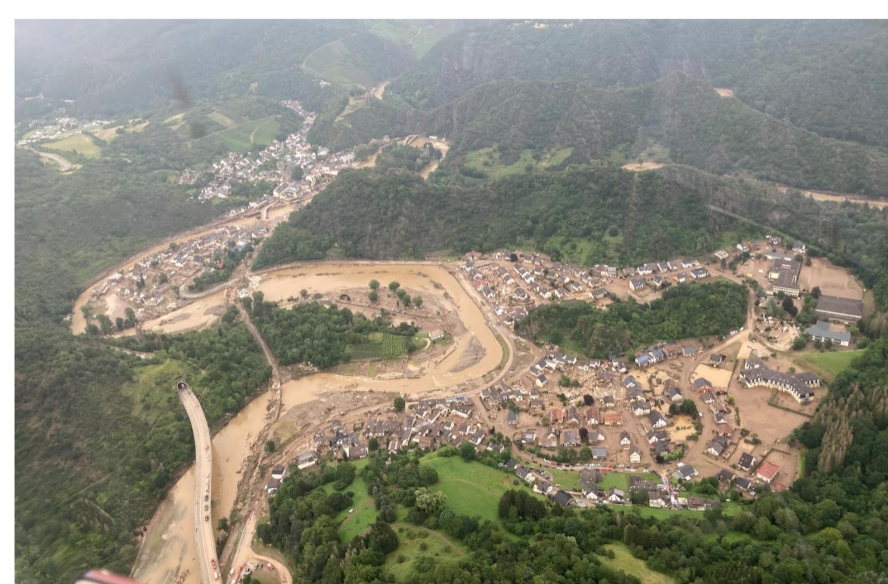
Damages along the river Ahr from 16 July 2021
