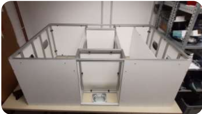
Cladding the walls with Trespa-plates
