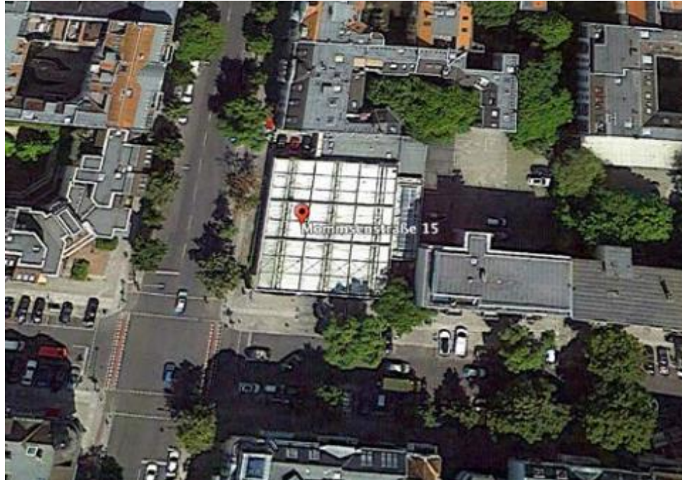
Figure 28: Former petrol station rededicated in 2019; date: 07/2012; Source: Google (2024)
