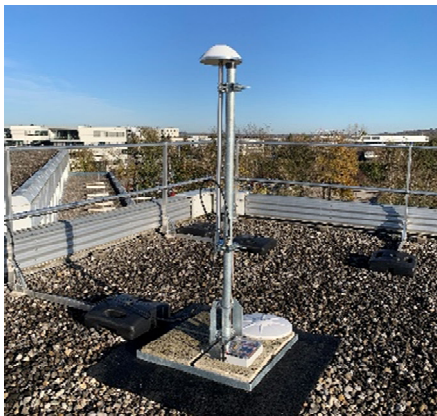
Fig. 12. Nose sub-assembly mock-up during the roof-top test performed to assess the impact of the anti-static paint onto the receiving performance of the GNSS antenna element.
