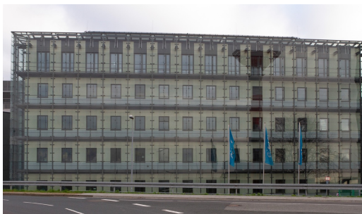
(a) AWI Building - Real
