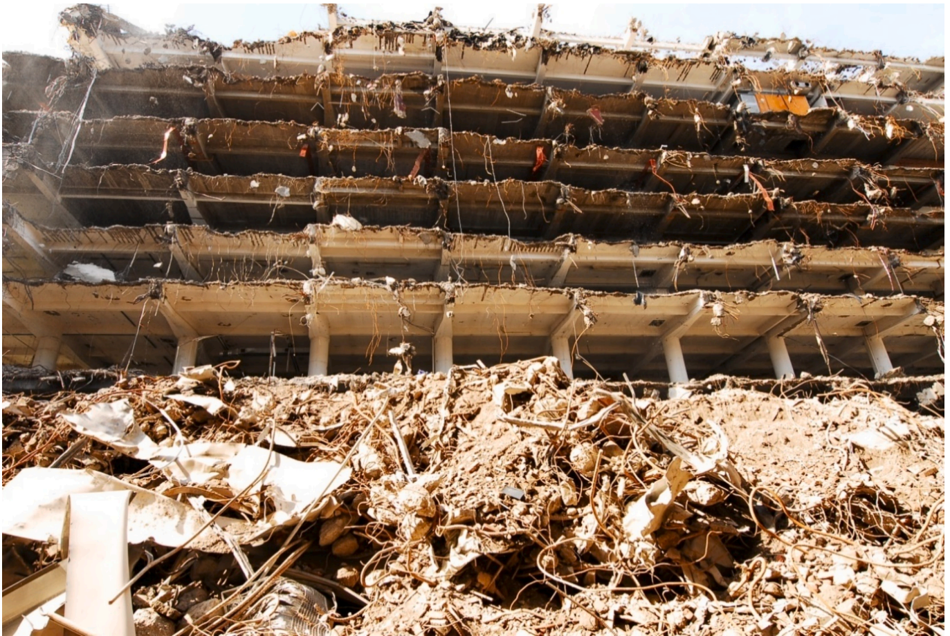
Fig. 3. Demolition in Brussels. Source: author's personal archive.
