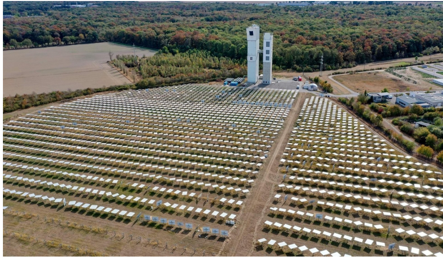
Figure 2.4: The solar tower plant in Jülich. The left tower holds the receiver as well as the power conversion system. The right tower is used for research purposes and is not part of the power plant (DLR, n.d.).
