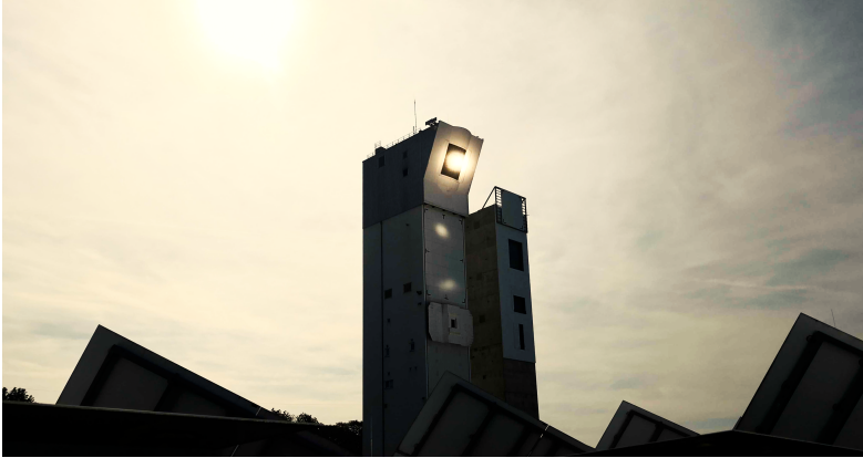
Figure 3: Image of the solar tower in Jülich from a view point inside of the heliostat field. While the majority of the heliostats is focusing on the receiver, two heliostats are calibrated simultaneously at an area below that.
