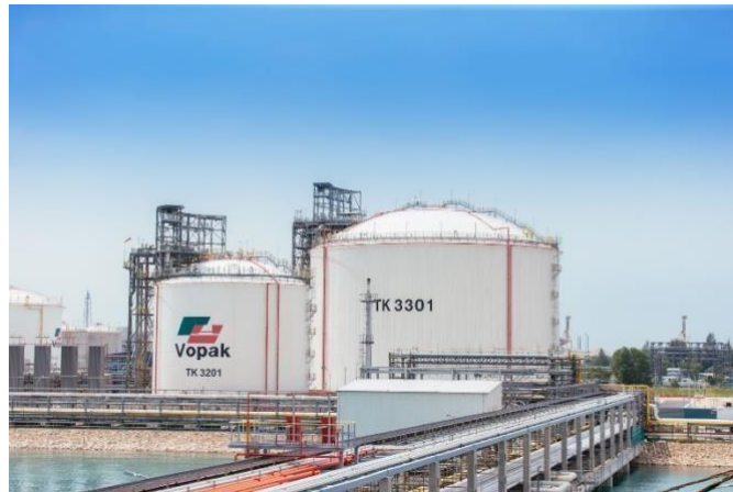
Figure 3- REPRESENTING THE VERTICAL TANKS FOR STORING FUELS IN OFFSHORE/ONSHORE PLATFORM (vopak)
