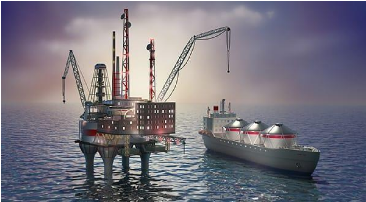
Figure 7- DEPICTS THE METHOD OF TRANSFERRING THE FUELS FROM OFFSHORE PLATFORM TO TANKER VESSEL USING PIPE AND PUMP SYSTEM (RBN)
