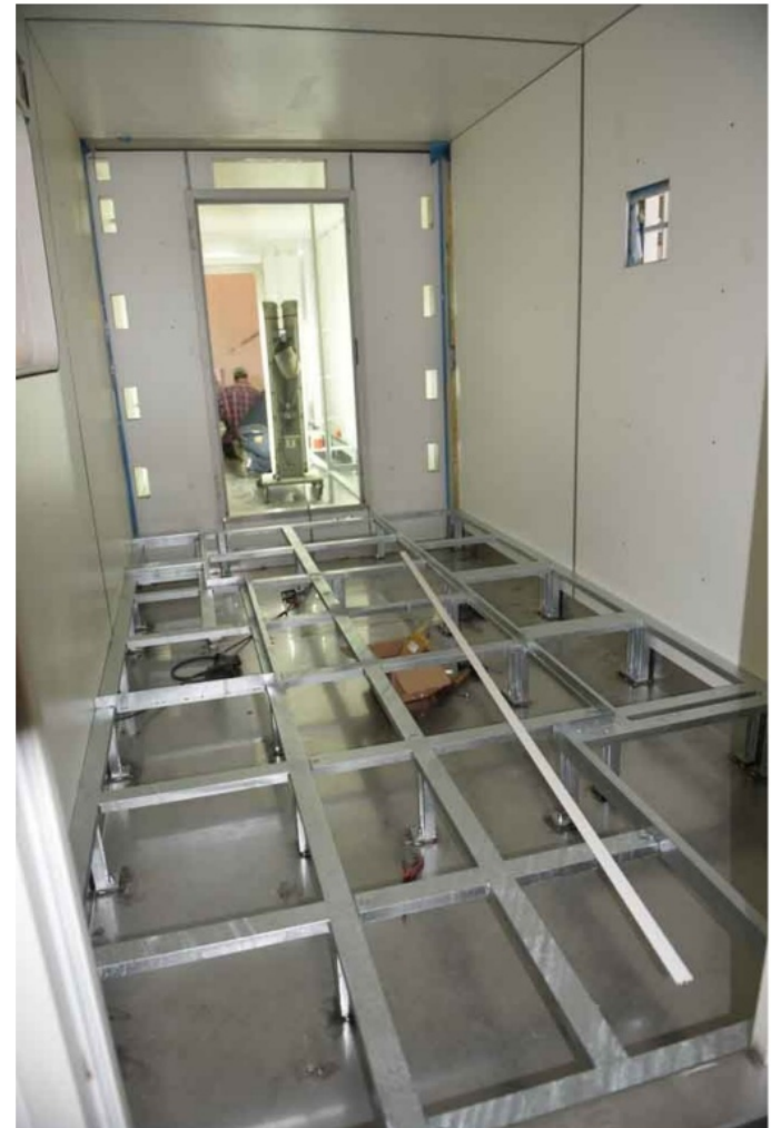
Internal sub floor structure of the FEG
