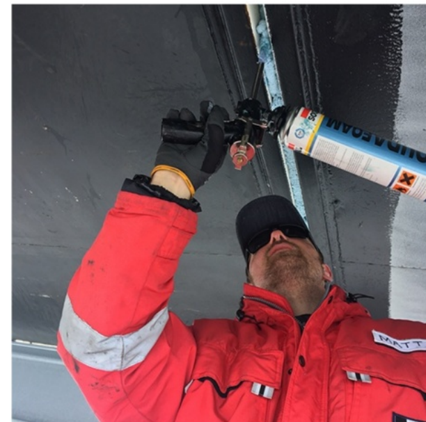
Thermal insulation between the two containers
