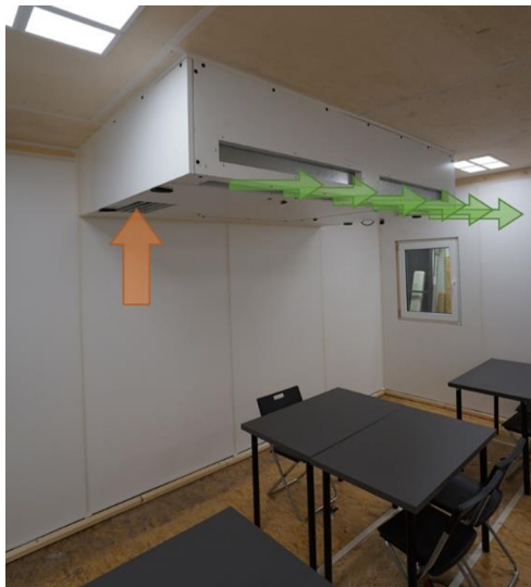
Fig. 5. Photo of the installed ceiling-based unit with arrows highlighting the induced air flow.
