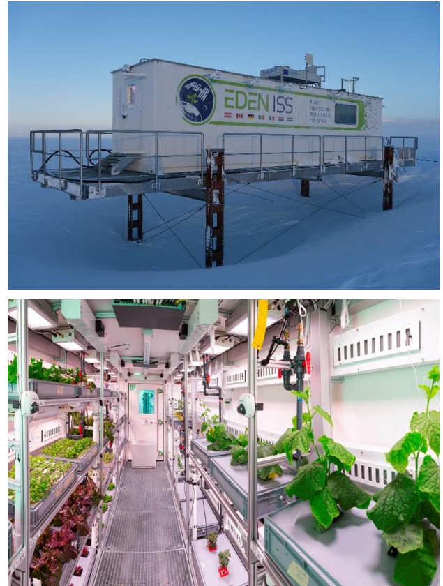
Figure 1. The EDEN ISS MTF as operated in Antarctica (top), consisting of two 20-foot containers – one acting as service section and one as greenhouse (bottom) with an aeroponic nutrient delivery system.
