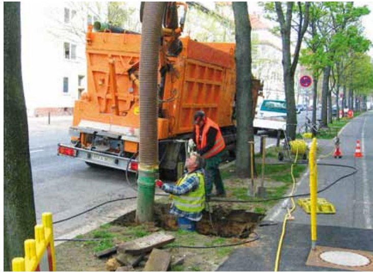
Figure 2. Site restoration of street tree in Hannover. Taken from Hannover Division of Environmental Protection (2017).
