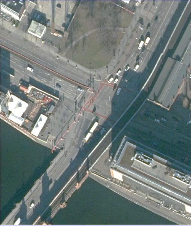
Fig. 7 – Aerial view of Oberbaumbrücke/Mühlenstrasse (source Geoportal Berlin/DOP20RGBI).
