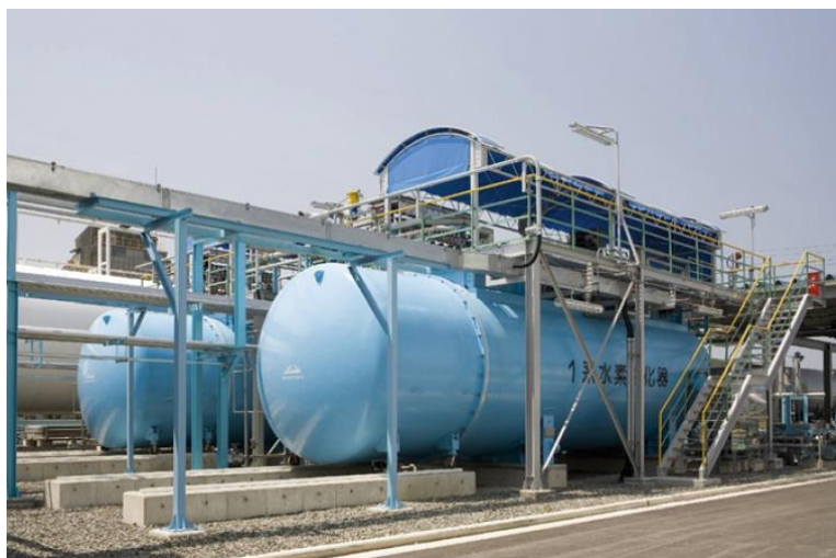
Figure 27: Hydrogen liquefier. (Courtesy of Linde Kryotechnik AG, Switzerland)
