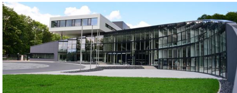
FIGURE 1.2. DLR Lampoldshausen front office and museum [26]
