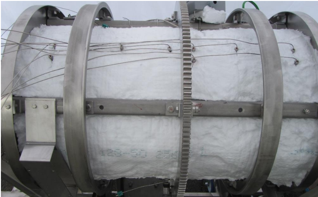
Figure 3.11 Reactor with second layer of insulation material
