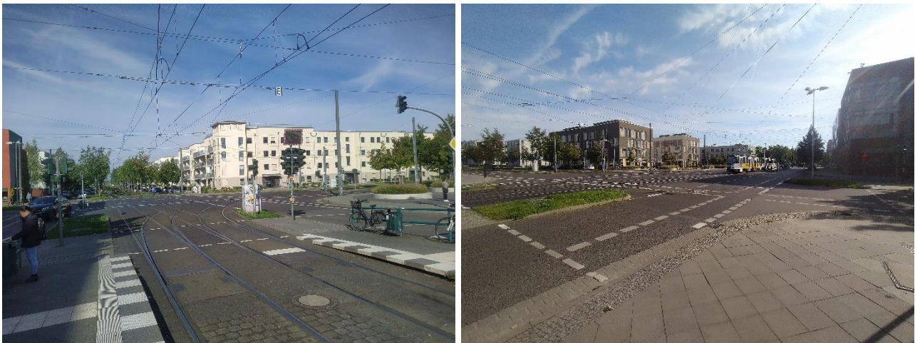
Figure 2: Living lab 2 – test intersection with traffic lights
