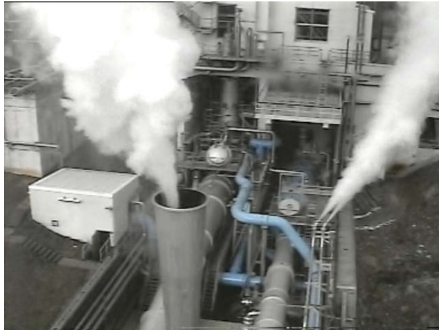
Steam ejection of the main ejector stages (left) and at the vacuum gate valve location (right) during dynamic vacuum test at P4.2
