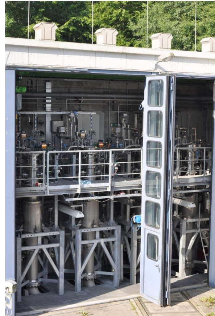
Four large steam generators
