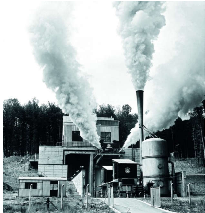
High Altitude Test with own development of steam generators and Astris engine at P4
