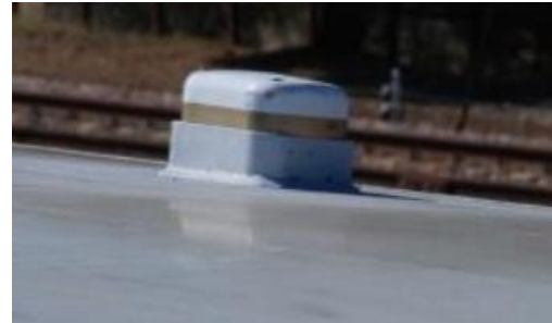
Figure 4. Antenna installation, Spain.
