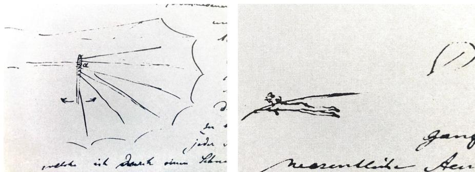
**Fig. 3** Illustration of Lilienthal's wing warping mechanism (left) and the extreme pilot posture required (right) to counteract a diving flight attitude with weight shift control as sketched and described only in a letter (reprinted in part from O. Lilienthal: Letter to A. Wolfmüller, 1895/10/03, © archive Deutsches Museum München, Acc. 1932-1/11 source [15]; <https://lilienthal-museum.museumnet.eu/archiv/objekt/15904>).
