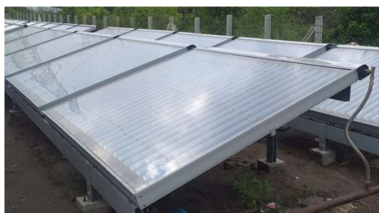
FIGURE 1. CPC collector ETC-CPC-24 with glass cover in NTPC solar field (photo: NTPC)
