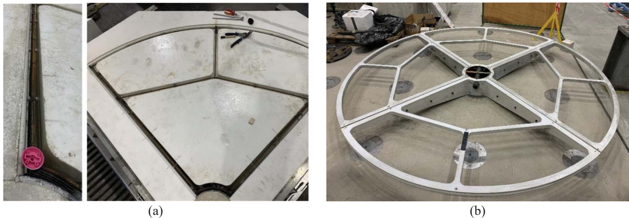
FIGURE 7. (a) Modular polystyrene formwork with reinforcement detail, (b) concrete modules connected to the inner steel ring
