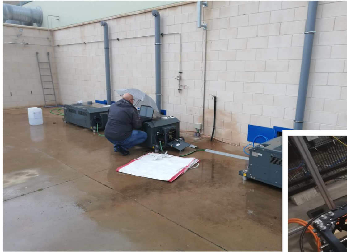
Cooling system connection/communication process (commissioning)
