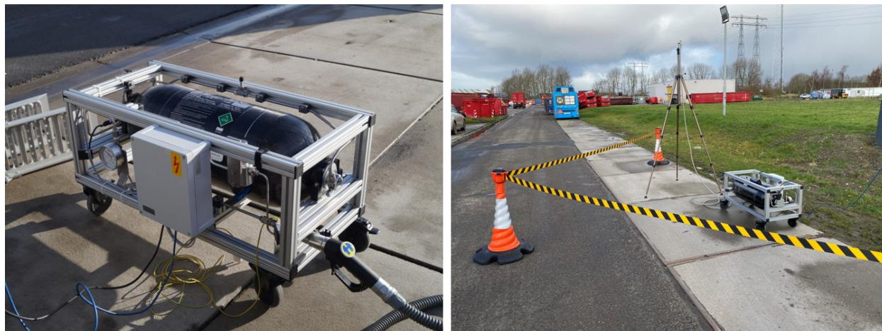
Figure 3. Visualization of hydrogen sampling for contamination analysis using the mobile tank. Shown are the refueling at the HRS and the venting of the hydrogen for purging near the refueling station with the barricaded work area.
