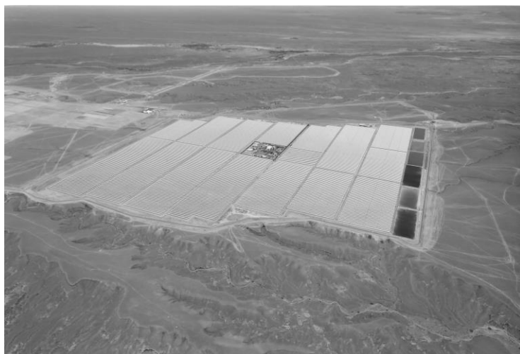
Figure 5. Steam cycle power station and solar heat storage in the center of the concentrating solar thermal collector field of NOOR 1, a CSP plant with 160 megawatt power capacity at Ouarzazate, Morocco commissioned in early 2016.
