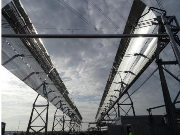
**FIGURE 3.** Parabolic trough collectors for steam generation at ADPO plant in Belgium
