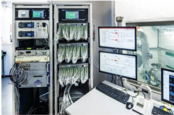
Hundreds of sensors deliver data to the measurement system of the ICD test rig
