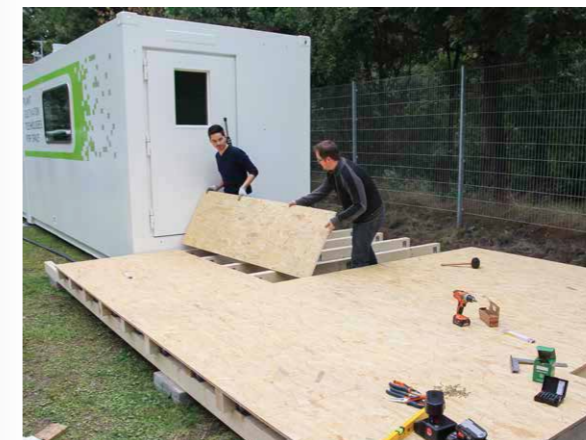
Construction of the AIT tent platform
