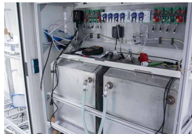
Partially installed EDEN ISS nutrient delivery system
