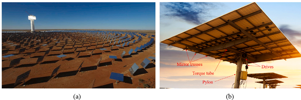
Fig. 1. Photographs of (a) the 50 MW Khi Solar One heliostat field (Abengoa Solar 2016), and (b) structural heliostat components of the Abengoa Solar heliostat. Adapted from Advisian Worley Group (2021).
