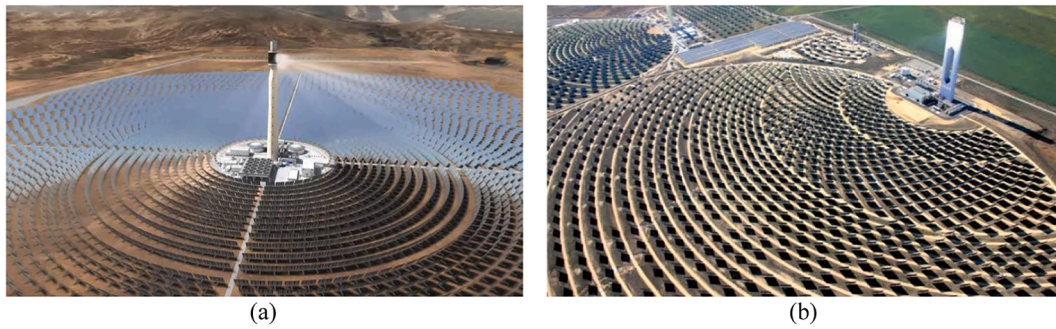
Fig. 22. Different layouts of a heliostat field. (a) A radial heliostat field, Noor III in Morocco. Image from www.masen.ma , (b) a polar heliostat field, PS10 in Spain. Image from www.eusolaris.eu .
