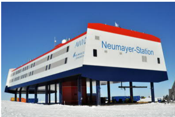
Fig.1 Neumayer-Station III. (© Ude Cieluch, Alfred-Wegener-Institut, retrieved on 2010 from www.daburna.de ).
