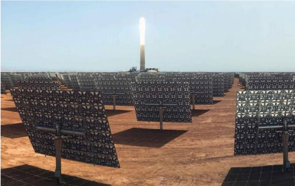
SENER's Heliostats at Noor 3 plant in Ouarzazate
