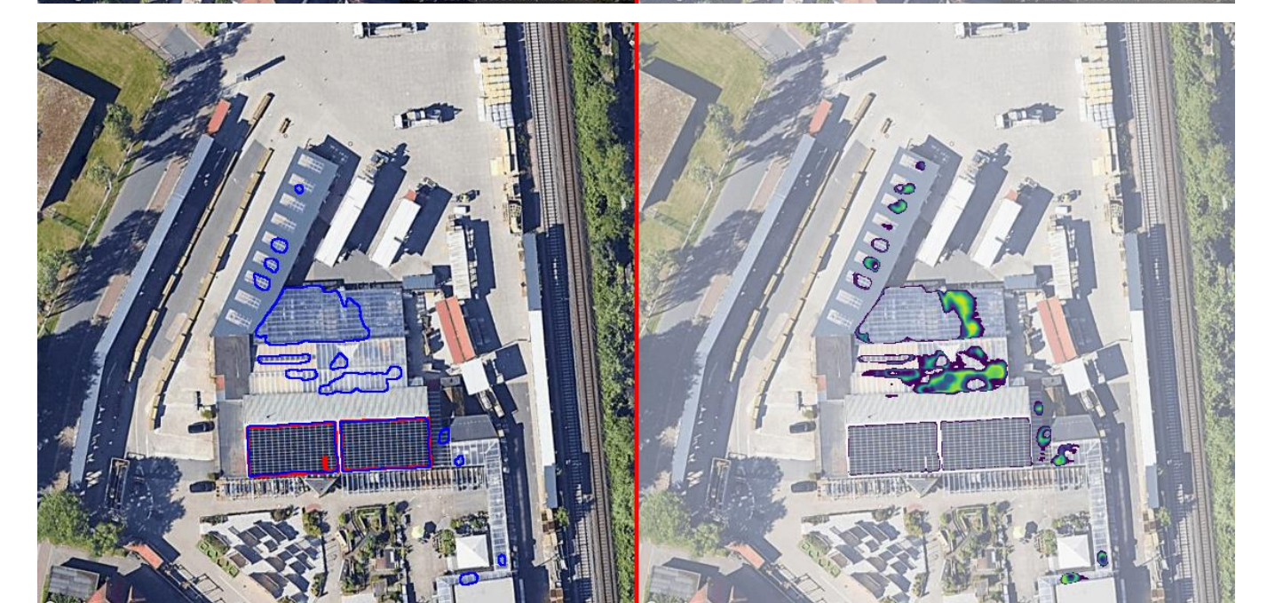
Primary rooftop system identified well, but false positives on glass rooftop and skylights. Uncertainty is high for the false positives, indicating potential for deeper look at uncertain cases.
