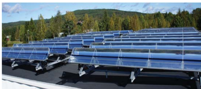
FIGURE 7. Parabolic trough collectors with glass cover on rooftop (photo Absolicon)
