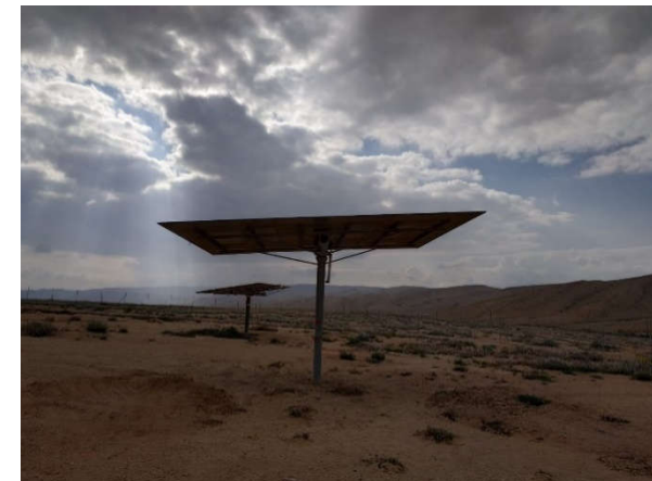
Thin-glass composite heliostat at BSII, Israel, erected autumn 2018
