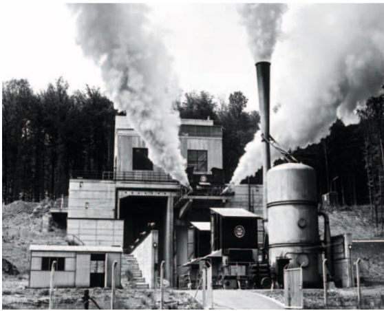
Fig. 5. P4 during a hot-fire vacuum test of “Astris”
