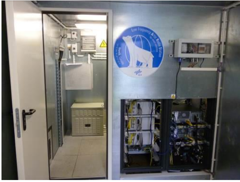
Fig 2. View from the working area into the utility room
