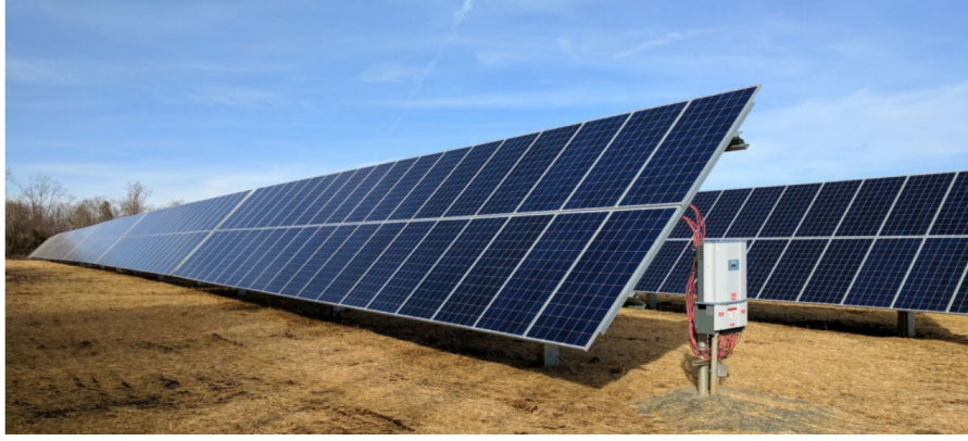
Figure 14: Single Axis Tracker with 2 in Portrait Configuration [6]
