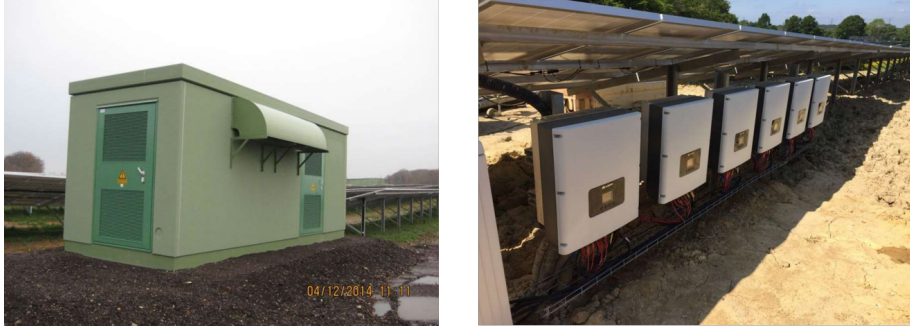
Figure 4: Centralized inverter (left) and string inverters (right) [6]
