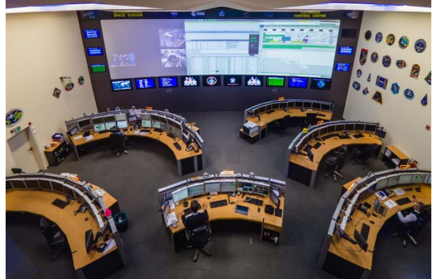
Fig. 2: Col-CC Main Control Room (Photo: Zoeschinger)
