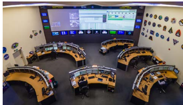
Fig. 3: Main Control-Room K4 at Col-CC (Photo: Zoeschinger)
