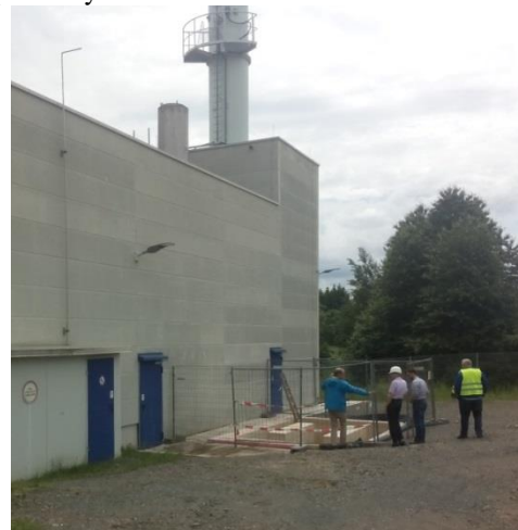
Figure 11: Foundation for the storage unit prepared for storage erection.
