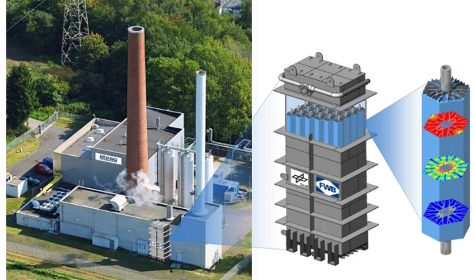
Figure 10: Photomontage of the storage unit erected along the wall of the cogeneration plant in Saarland, Germany.
