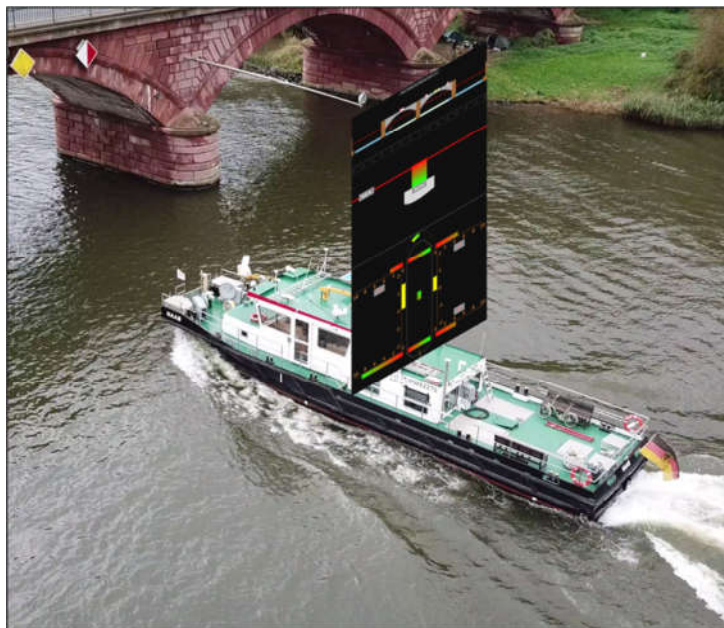
Figure 1: Bridge collision warning system
