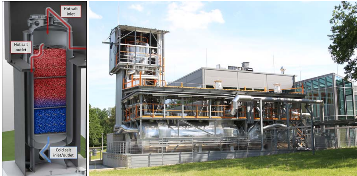
Fig. 2: Illustration of the thermocline filler storage tank of the TESIS facility (left) and picture of the plant (right)
