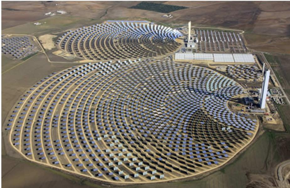
**Figure 2.3** Two CSP tower plants in Spain (PS10 and PS20) [53].
