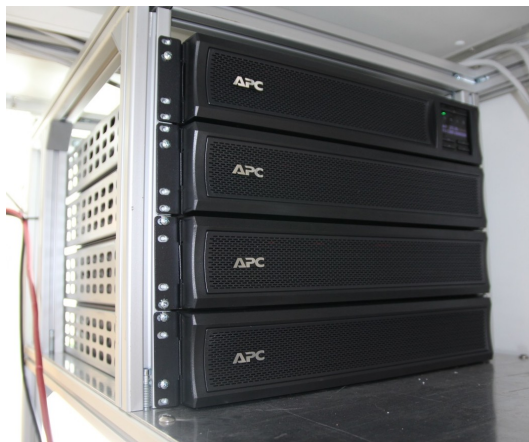
Figure 6: UPS mounted in the top compartment of the NDS rack. Credit: DLR
