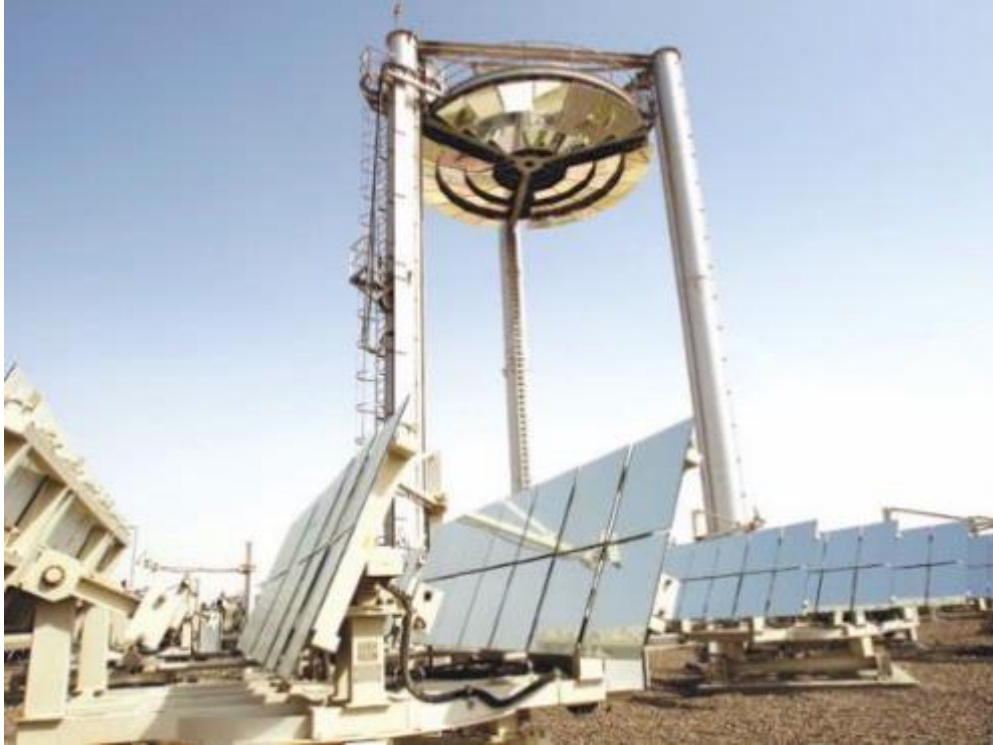
Heliostat field and Beam-Down Tower at the Masdar Institute Solar Platform (MISP)
