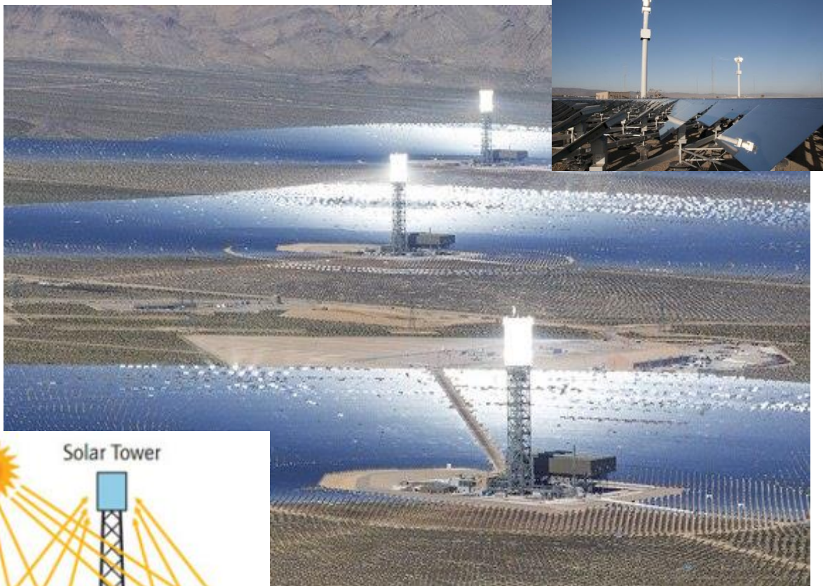
Ivanpah 392 MW - Solar Tower
