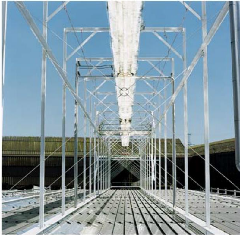
Figure A-45: Energy production above and horticulture underneath a linear Fresnel collector field in a multipurpose concentrating solar thermal power plant. Photos of the collector field by Solarmundo, greenhouse visualisation by DLR.
