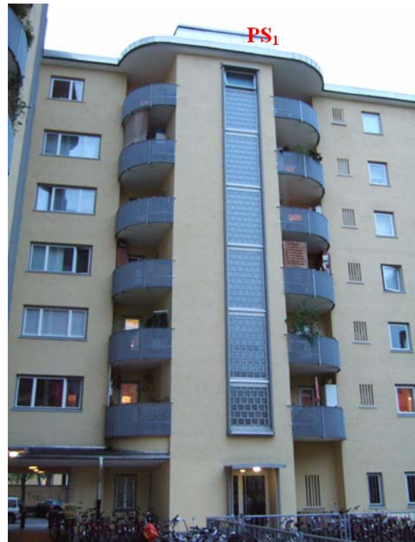
Figure 11: Photo of the first of the two scatterers which are located in one and the same resolution cell. This building is the PS1 and has a height of about 25 m. Figure 12 describes the second scatterer.
