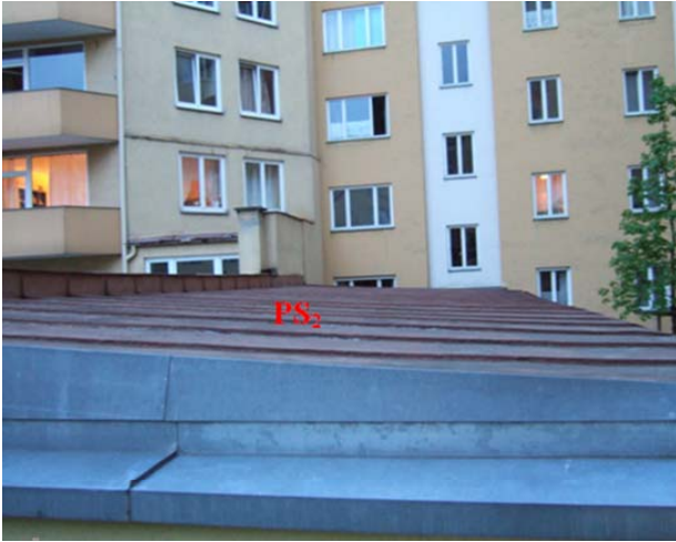
Figure 12: Photo of the second of the two scatterers which are located in one and the same resolution cell. The roof made of metal is the PS2 and has a height of about 2 m. Both scatterers are separated by about 64 m in ground distance causing both to appear in one and the same resolution cell. The developed parametric algorithm is able to detect this sort of resolution cell and to estimate the height separation of about 24 m between the two scatterers.
