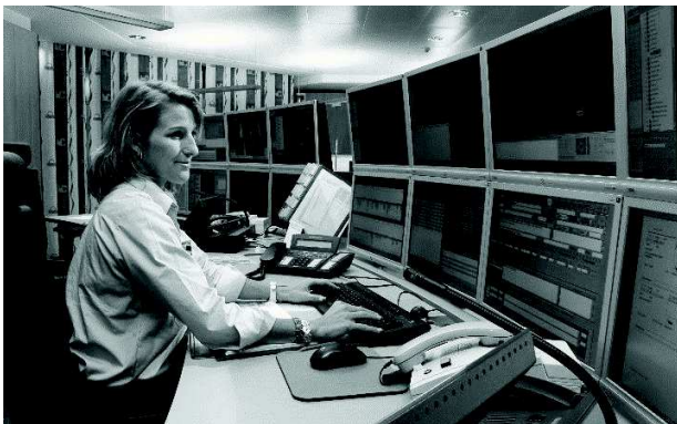
Figure 5. Operations control center
