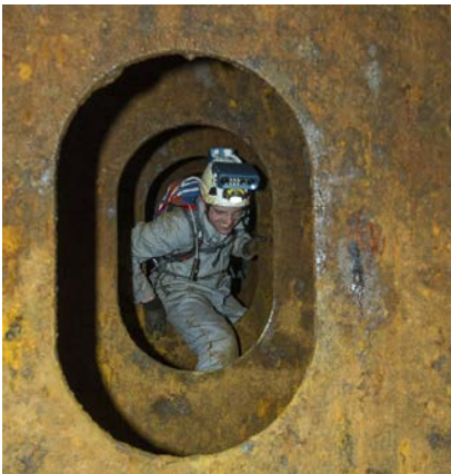
Figure 11: IPSpect in ballast water Tank 1
